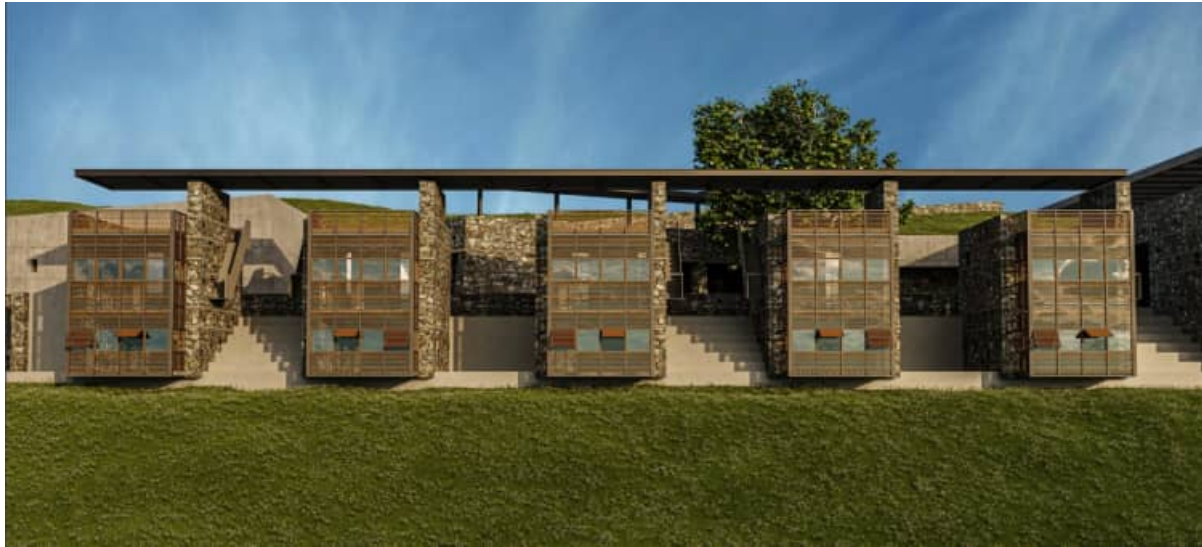
Picture 13: Front view
